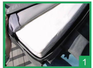
Heat sealed vapor wrap.
